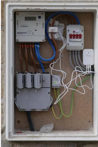
**Figure 4:** An 'Owl' system measuring EV charging stream.
